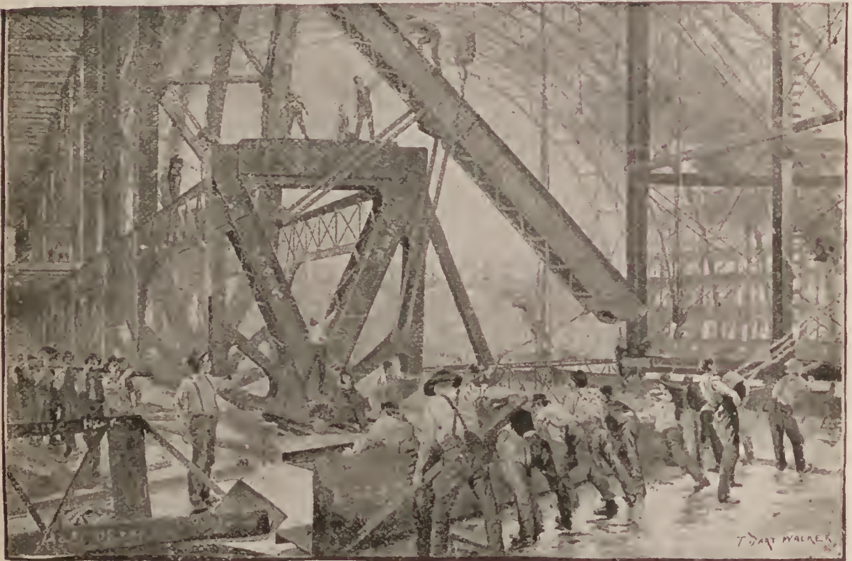
ERECTION OF MANUFACTURES BUILDING.
